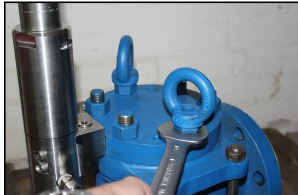
Figure 2: Unscrewing an eyelet
