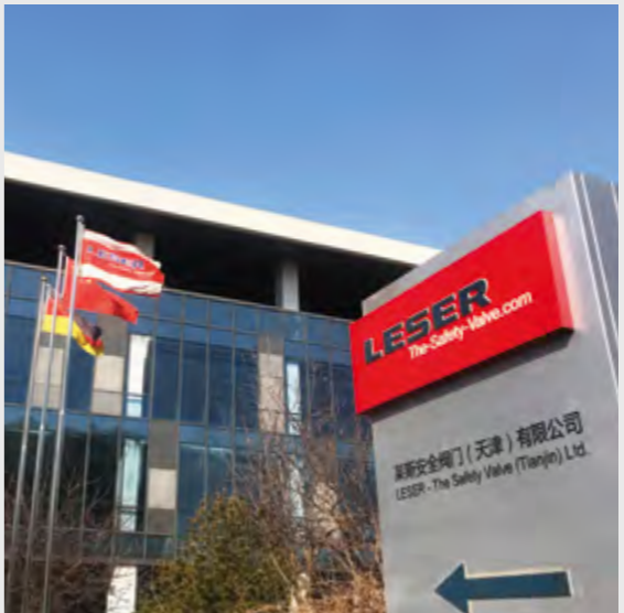
LESER China, Tianjin Manufacturing and Administration Site
